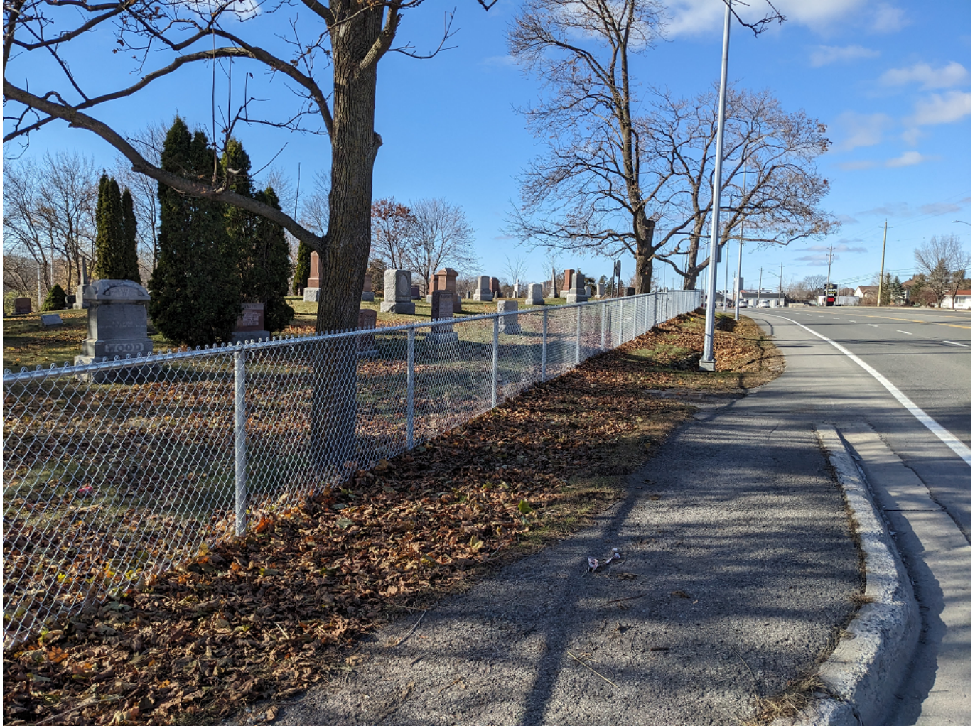
New Wood's Cemetery Fence Installed by McGee Fencing Ltd. in November 2023
